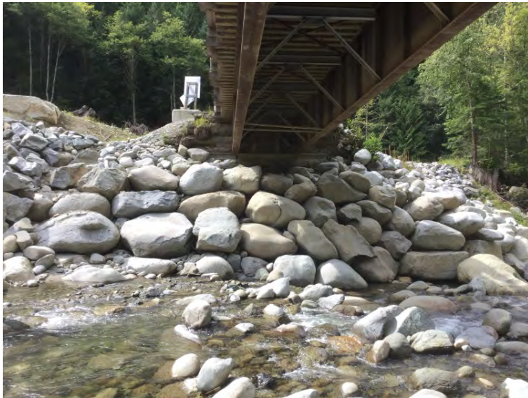
Left Bank Abutment when facing downstream
