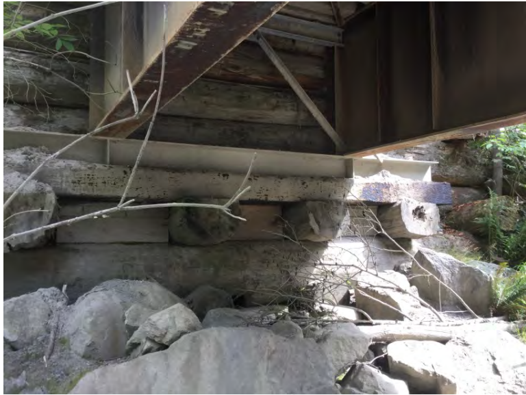
Right bank bearing
