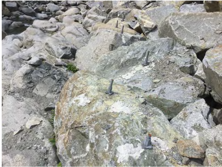
Riprap bolting upstream
