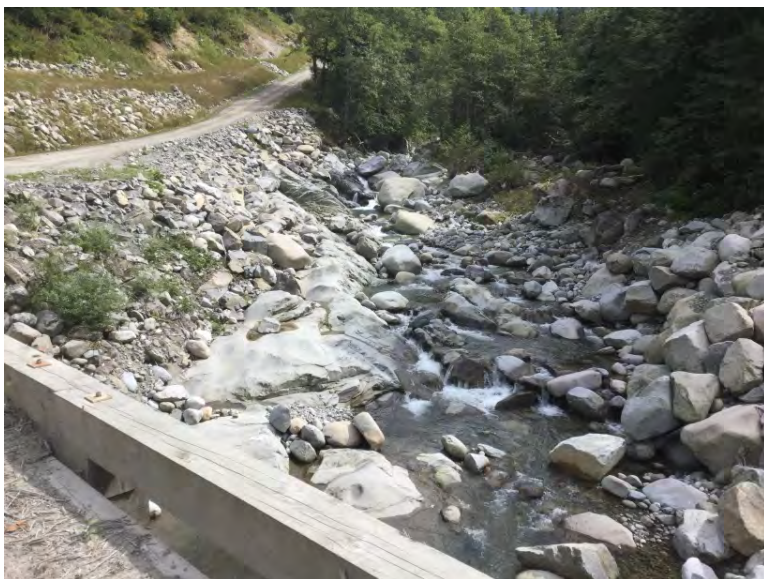
Upstream from Crossing
