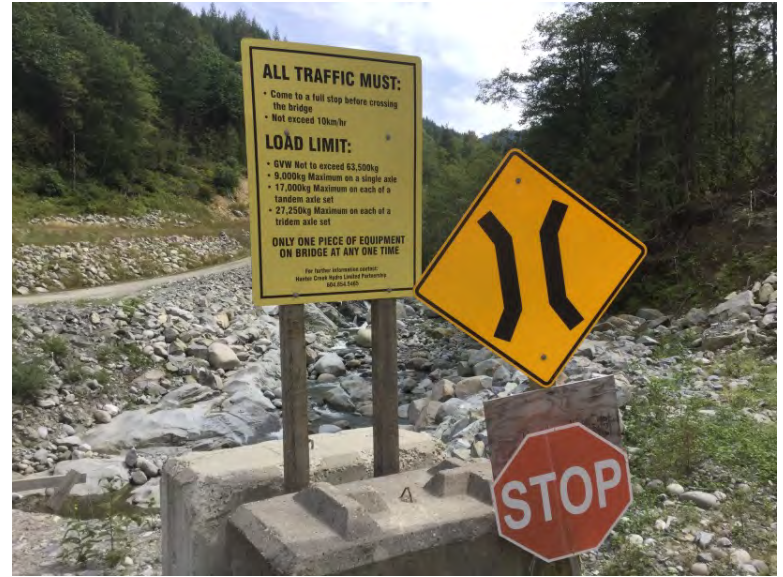
Load Rating Sign
