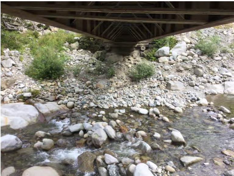
Right Bank Abutment when facing downstream
